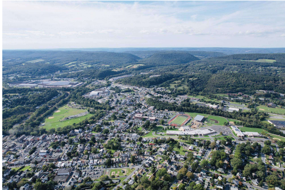
Photo: Liberty Haven Fire Company #4
